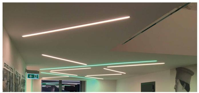
Decorated anodised aluminium lamp complete with brushed or microprismatic diffuser and high-brightness LED source with a high Lumen/Watt ratio. Suitable for primary residential, retail, large-space and general lighting. Flush-mounted
